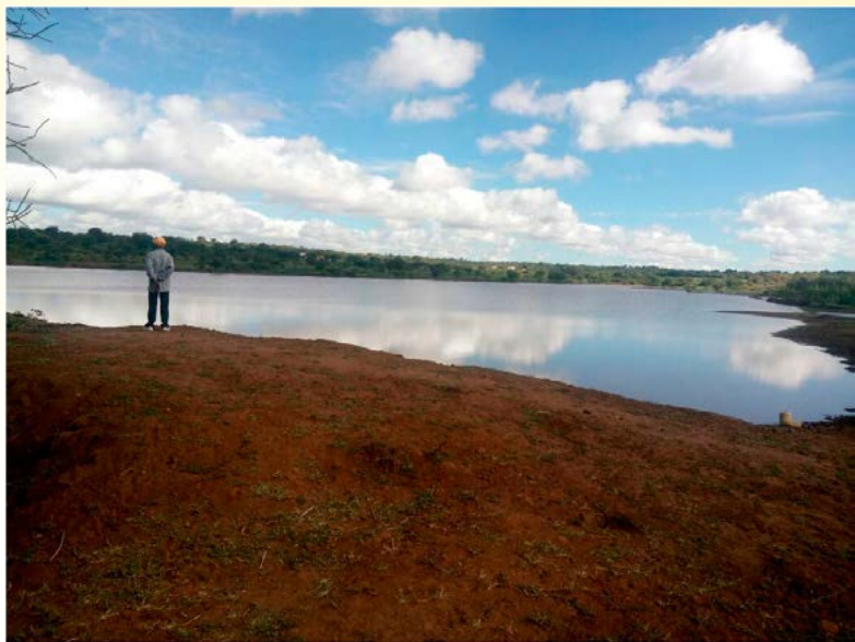
Mikuyuni Earth Dam in Kauwi ward, Kitui County
