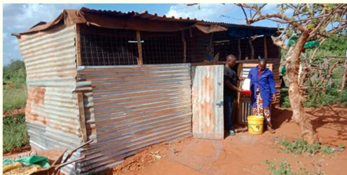
Mwende outside her locally constructed poultry house listening carefully as Nzuki-ADSE trains her on how to fix the water trough to ensure steady supply of water
