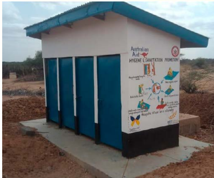
A VIP latrine constructed in Garissa
