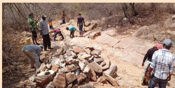
Community members in Katangi Ward mobilize local materials to support the construction of a sand dam that will enhance water availability. Photo by ADSE
